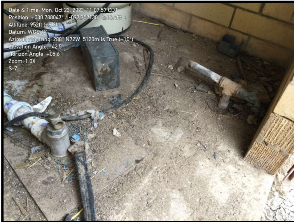
Groundwater wells S-7 (left) and S-12 (right).
