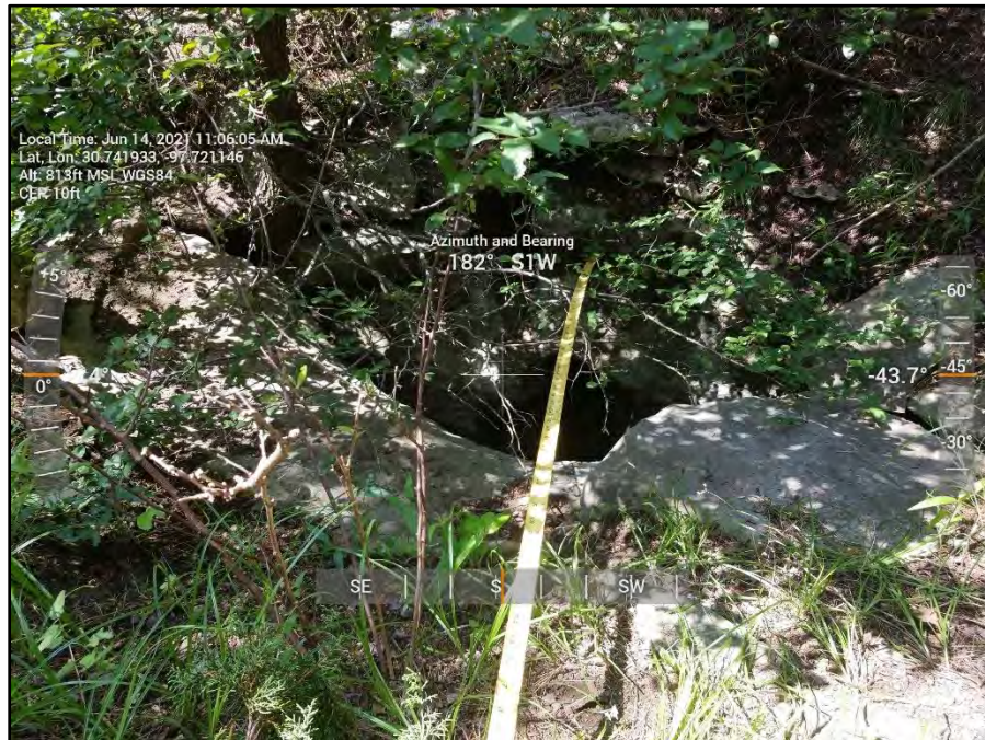
M-04 (View of depression)
