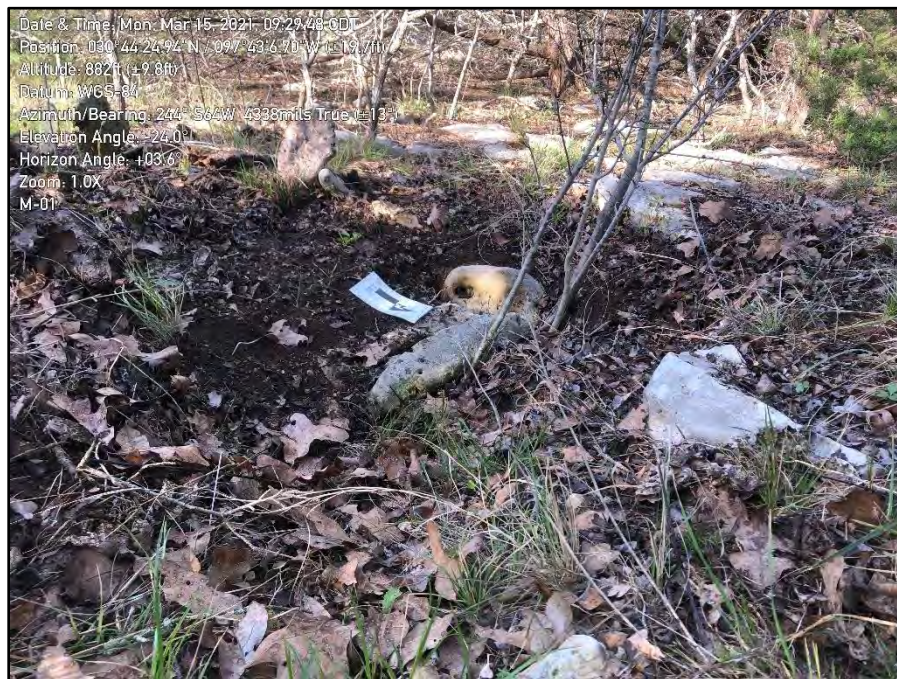
M-01 (view showing depression).
